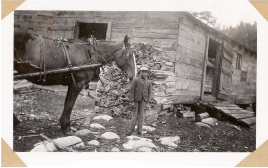
The Anderson saw mill and a pile of finished barrel staves behind the young boy. The horse and wagon are also owned by Mr. Anderson. On the other side of the mill there is a lake, the source of water power.
